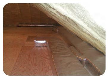
The supply trunk on the right replaced 3 excessively long flex run-outs.
