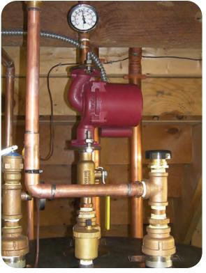
Triangle Tube lifetime-warranty, stainless steel indirect-fired water heater (left). My lead-free bronze circulator flanges connect to the Grundfos circulator for hot water re-circulation. Potable water connections (right) are on top, and boiler water connections (not shown) are in the back of the tank-within-a-tank.
