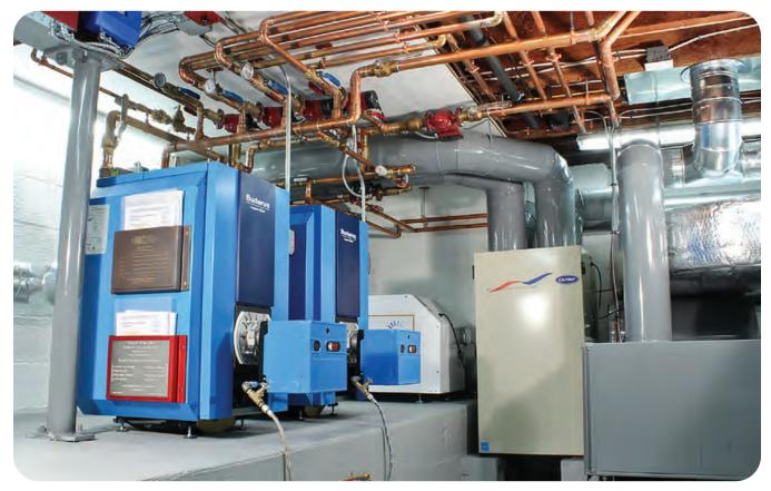
My document holder and valve handle inventions can be seen on the boiler and local piping. The Buderas cast iron boilers are oil-fired G215/3 models, and are controlled by a Tekmar staging/temperature modulation control.
