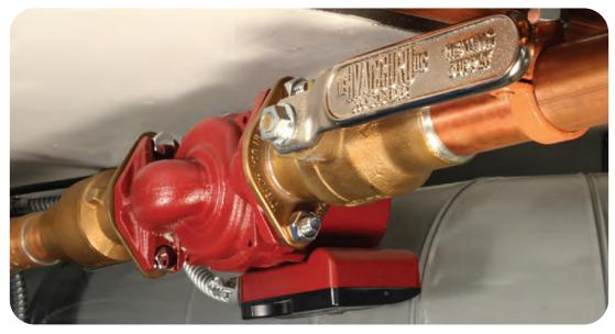
Nickel-plated bronze "Heating Supply" handles on  $1-\frac{1}{2}$ " valves that isolate the supply line to the Triangle Tube indirect-fired water heater.
