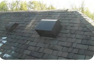
From top left, clockwise: 32-foot stainless steel Z-Flex chimney liner passes up through existing chimney; close-up of termination; whole house fan vent and master bath exhaust vent.
