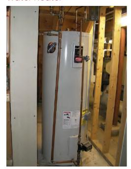
Not-energized electric water heater used as a storage tank, with plate-type heat exchanger (top right of center).
