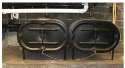
Sediment collected at the bottom of the dip in the oil line preventing oil from evenly draining from both tanks. The oil filter was installed, wrongly, just before the burner.
