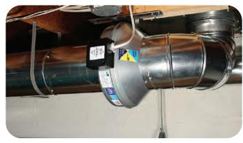
Two 600-CFM exhaust fans (identical to the master bath) for 1<sup>st</sup> floor baths were installed and vented through rim joists.
