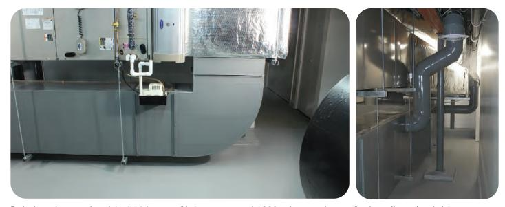
Painting ductwork added 16 hours of labor cost and \$200, plus or minus, of other direct/variable costs. The white diffuser (right image) delivers fresh air to the mechanical room. The same fresh air supply feeds the return plenum of the A/H.
