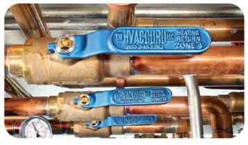
Red and blue anodized aluminum handles intuitively differentiate supply (hot) from return (cold) pipes.
