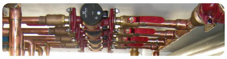
Grundfos Alpha circulators were chosen to maximize performance with the lowest electricity consumption.
