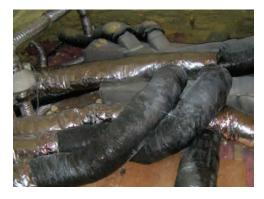
All of the "run-outs" in the attic were flex duct, and were kinked and excessively long.
