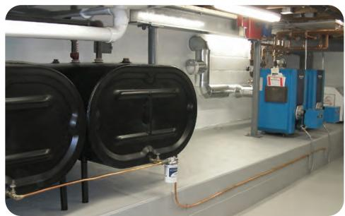
The dip in the oil line was eliminated, and a highly effective oil filter (Westwood F100) was installed on the outlet of the two-tank oil supply manifold. The 9" 24 gauge smokepipe connects to a 32-foot Z-Flex stainless steel chimney liner (see page 13). A new cleanout door was installed.
