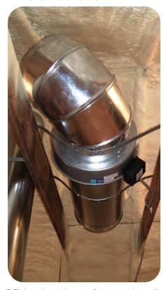
A 900-CFM attic exhaust fan was installed and vented through the roof (see page 13)-this acts as a whole-house fan and removes insulation "out-gas" odors from the attic.
