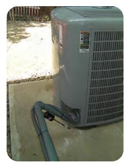
Two-speed Carrier condensing units match A/Hs to produce the highest SEER (efficiency) rating. A concrete pad was poured specifically for them. Pipe insulation was painted to shield it from degrading UV rays.
