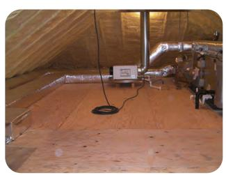
The space is now accessible without stepping on ducts, or mis-stepping on unfastened plywood, through the insulation and sheetrock ceiling below.
