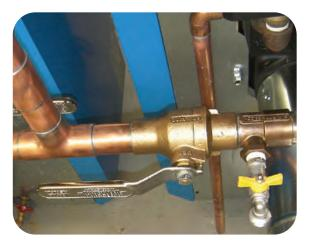
Like my bronze flanges, the  $1-\frac{1}{2}$ " Male (Street) X  $1-\frac{1}{2}$ " Female X  $\frac{1}{2}$ " IPS lead-free, bronze sweat (solderable) Tee eliminates the need for a length of copper pipe to join it to a valve or fitting.
