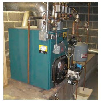
Each heating zone was controlled by a thermostat and zone valve. One circulator proved insufficient to supply hot boiler water to all zones simultaneously.
