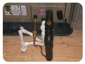
Valves on refrigerant lines and unions on condensate drains facilitate future maintenance.
