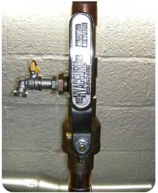
Tee is behind the nickel-plated, polished/buffed bronze 1-½" valve handle, and has a purge valve (yellow handle) attached.
